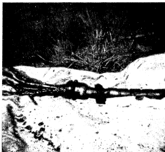
NO. 12.—PART OF CABLE-END BOX AND CABLE END AT SERVICE FUSE END.
