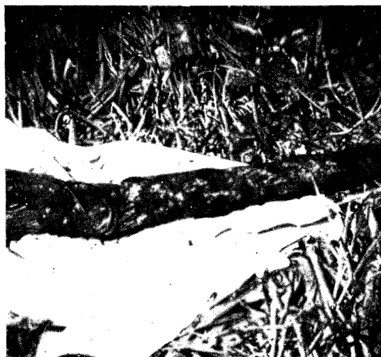
NO. 6.—FRACTURED CABLE 5 FT. 8 IN. FROM I BEARER END OF CABLE BREAK SHOWING DOUBLE STEEL TAPE ARMOURING SUBSEQUENTLY REMOVED IN COURSE OF EXAMINATION.
